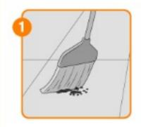
Clean the floor/wall surface to remove dust, oil & grease etc. properly so that there is no hindrance in adhesion.
