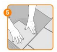
Ensure that the tiles are fully supported by adhesive. Apply adhesive at back of tiles, if required to accommodate level.
