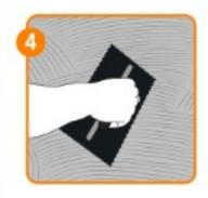
Apply the mix on the floor/wall surface in appropriate thickness using a trowel. 2mm bed thickness for wall and 3 mm for floor must be kept.
